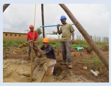
• Training in manual drilling in Mzuzu (August, 2 weeks). Trainer Laban Kaduma has travelled to Malawi to assist the SMART Centre in Mzuzu in giving training in drilling of wells using SHIPO method.
